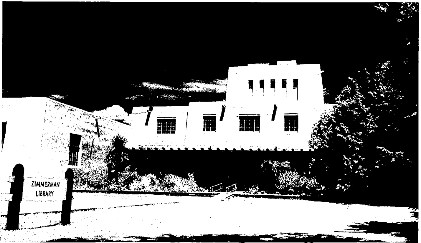
Zimmerman Library, west facade
