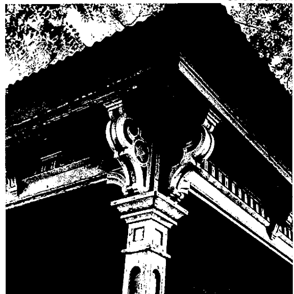
Porch support, Railroad Superintendent's House photograph by Christopher Wilson
