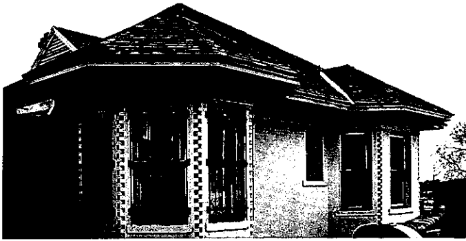
The second story of the Springer House photograph by Christopher Wilson
