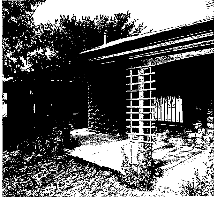
The Salvador Armijo House showing the cast stone facing on the south wing
