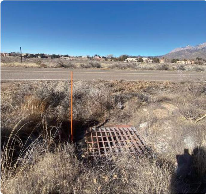
*Figure 9. Existing 24" RCP Outlets on North Side of Simms Park Road*
