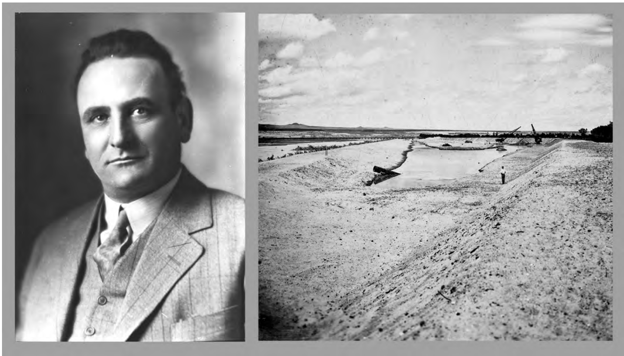
Clyde Tingley circa 1925, soon after becoming city commissioner. Tingley's direct plea to the newly-formed Middle Rio Grande Conservancy District led to the dredging of a lake along the river, as Aldo Leopold had first suggested. Right, cranes excavating Conservancy Beach in the summer of 1931.
