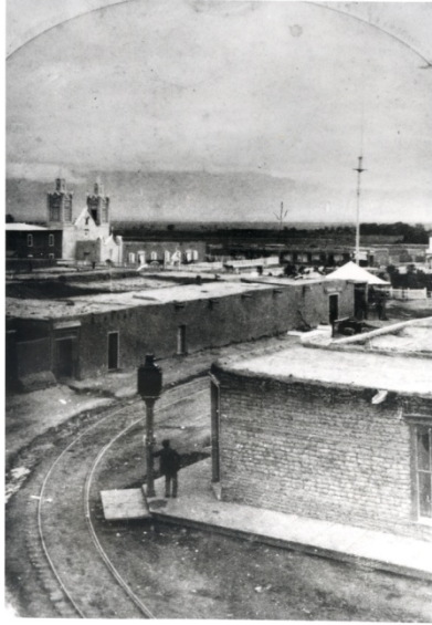
View NE Along Main Street, Now Rio Grande Boulevard - 1876
