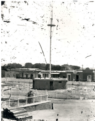
Plaza Guard House and Flagpole
