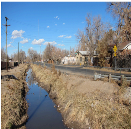
Alameda Drain South of Central Avenue
