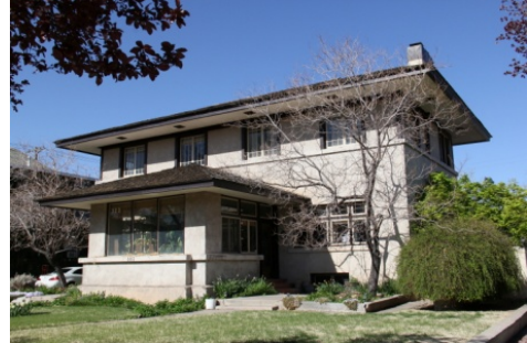
Berthold Spitz House - 323 Tenth Street NW – ca. 1910 – Prairie School Influence Is Apparent
