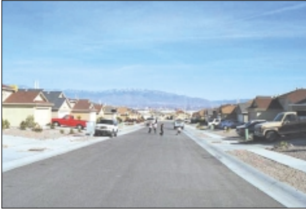
New Residential Development — Atrisco Area
